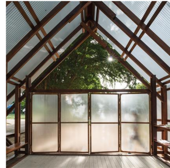
SHARED SPACE COULD BE LIGHTWEIGHT CONSTRUCTION AND FEEL MORE OPEN WITH FRAMED CONSTRUCTION AND A TRANSLUCENT LINING TO WALLS AND ROOF
