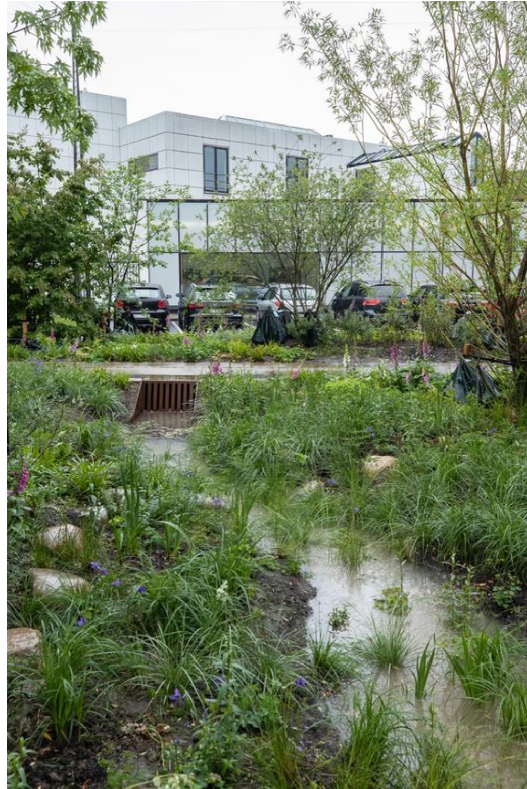
BIOSWALE IN LOW SECTION OF THE SITE WITH NATIVE PLANTING AND ROCKS. BIOSWALE WILL STORE AND FILTER RUNOFF AND DRAINAGE FROM BUILDINGS. AFTER TREATMENT THE WATER IS STORED IN AN UNDERGROUND TANK FOR GARDEN IRRIGATION
