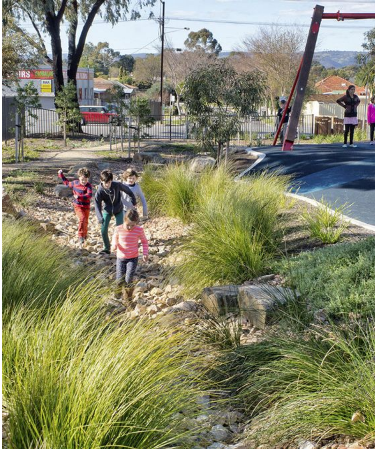
BIOSWALE IN LOW SECTION OF THE SITE WITH NATIVE PLANTING AND ROCKS. BIOSWALE WILL STORE AND FILTER RUNOFF AND DRAINAGE FROM BUILDINGS. AFTER TREATMENT THE WATER IS STORED IN AN UNDERGROUND TANK FOR GARDEN IRRIGATION
