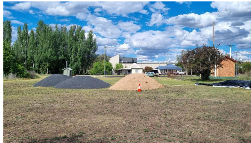
PHOTO 2: LOOKING NORTH EAST TOWARDS FRONT BOUNDARY. WOOLWORTHS IN THE BACKGROUND AND COUNCIL SEWER PUMP STATION TO SOUTH EAST
