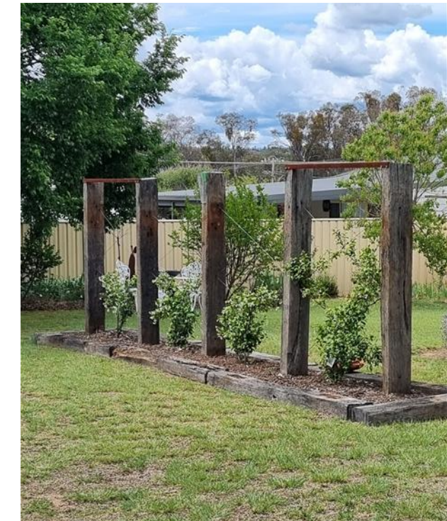
GROW STRUCTURES, THIS ONE IN LITTLE TIMOR STREET, COONABARABRAN. USE RECYCLED MATERIALS WHERE POSSIBLE
